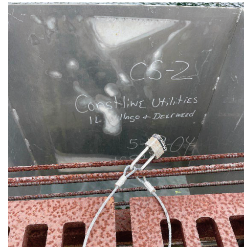
Lake 2 overflow structure.
