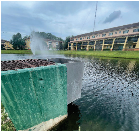
Lake 2 overflow structure.
