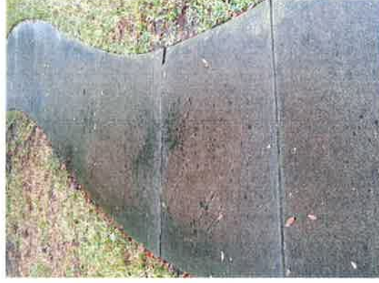
51-Cracking of Sidewalk
