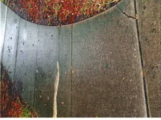
51-Cracking of Sidewalk
