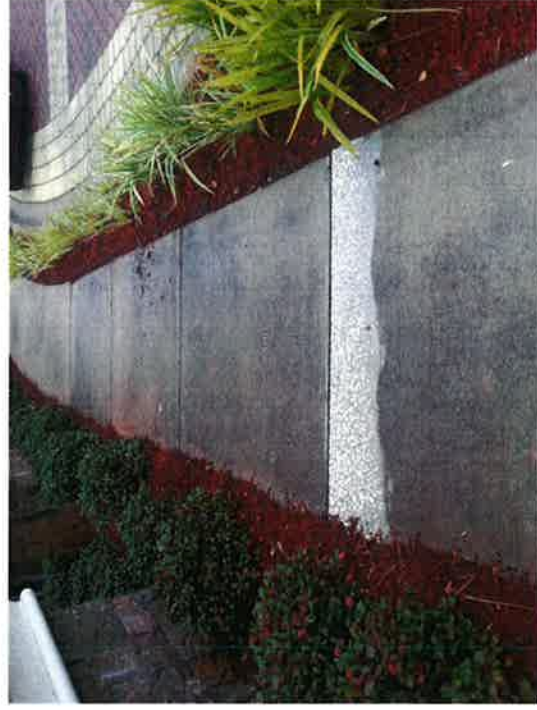
47-Grinding of sidewalk to eliminate deflection
