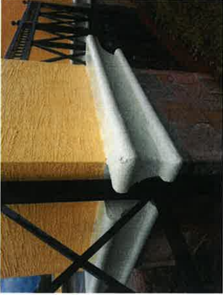
23-Peeling paint and bubbling at corner
