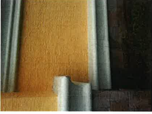
24- Peeling paint and vertical Crack
