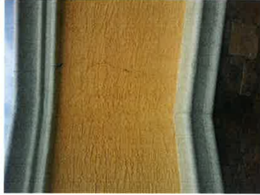
23-Peeling paint and bubbling at corner
